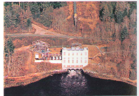
Lois Lake Generating Station
