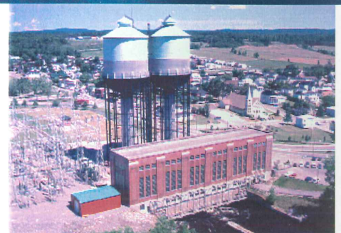
Masson Generating Station
