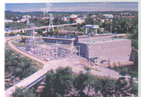
Dufferin Generating Station
